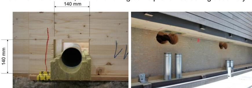
**FIGURE 8:** LEFT: DETAIL OF A VENTILATION DUCT DURING PRODUCTION OF THE FAÇADE MODULES IN THE FACTORY
