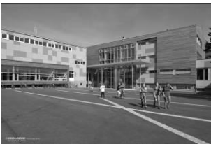
FIGURE 16: AFTER THE RENOVATION
