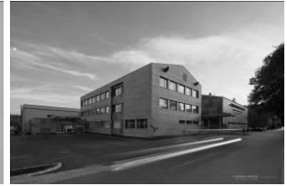
FIGURE 21: NORTH EAST SIDE
